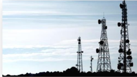
Ground Based Tower
