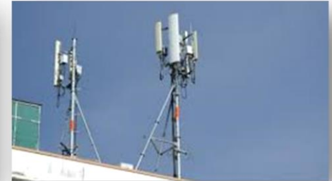
Roof Top Tower
